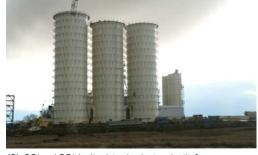
(3) 38' x 128' bolted tanks being built for a transload facility each storing 5,000 tons of sand.
