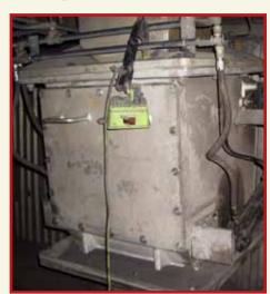
Generating Station, which is part of Integrys Energy Services. "Because the type of coal we burn puts added stress on the crushers in our fuel system, we take one of our two fuel lines down every three weeks to replace the hammers in the crushers."
